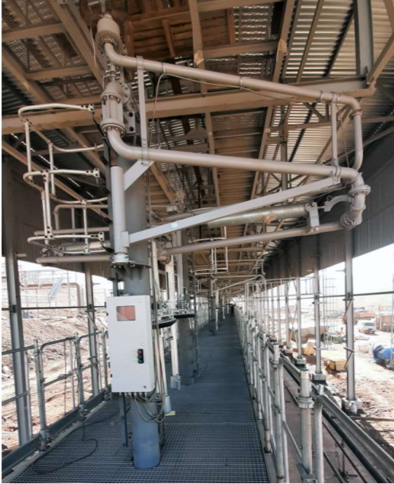
S-14ZHD-K Loading standpipe with a telescopic nozzle
